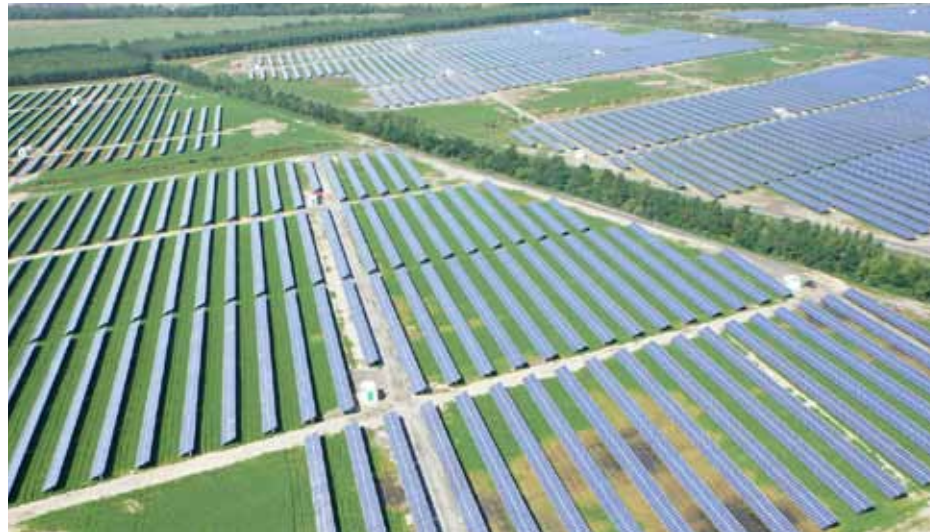
82MW ground-mounted installation in Senftenberg (Germany)
