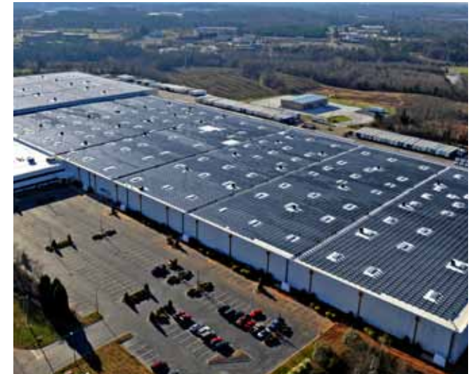
5.2MW rooftop installation in North Carolina (USA)
